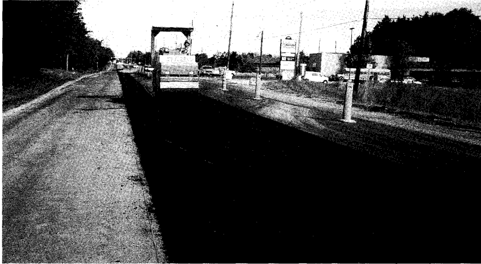
PHOTOGRAPH 5. Compacting the Surface Course Asphalt Rubber (AR) Hot-Mix Asphalt (HL 3AR) on Park Road North.
