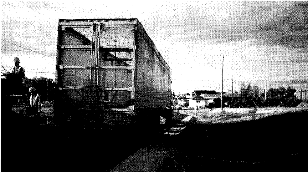
PHOTOGRAPH 10. Heavy Truck on the Just Compacted Binder Course Rubber Modified Hot-Mix Asphalt (HL 4MRUAC) on Main Street.
