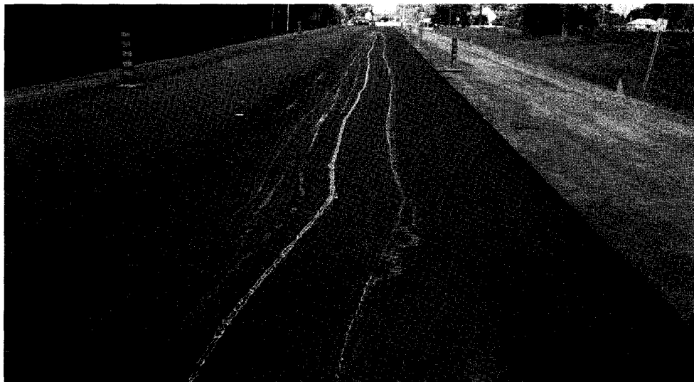
PHOTOGRAPH 6. Completed Surface Course Asphalt Rubber (AR) Hot-Mix Asphalt (HL 3AR) on Park Road North.
