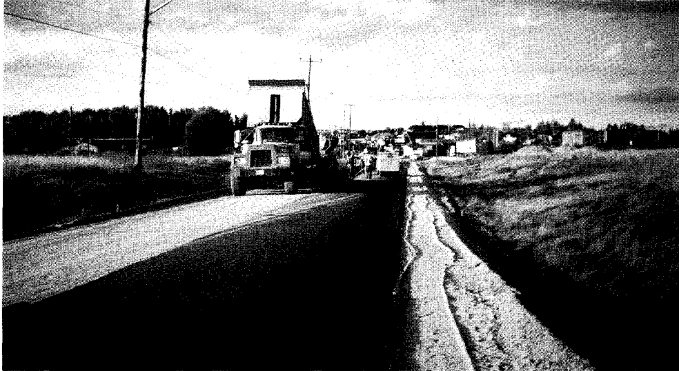
PHOTOGRAPH 9. Placing and Compacting the Binder Course Rubber Modified Hot-Mix Asphalt (HL 4MRUAC) on Main Street.
