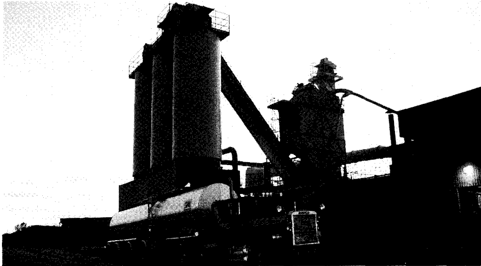
PHOTOGRAPH 3. Combined Drum Mixer/Batch Plant that Produced the Asphalt Rubber (AR) Hot-Mix Asphalt for City of Brantford Project.
